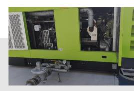
Bio-methane feed to the Pramac's Gas Power Generator set
